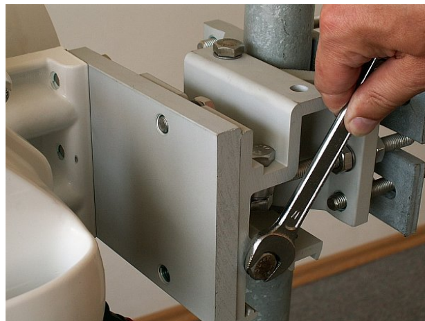
Fig. 5.17: Vertical adjustment of the antenna direction
