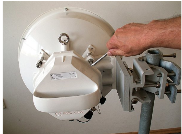
Fig. 5.15: Tightening bolts on the FOD unit
